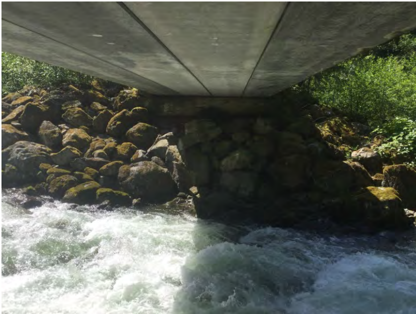
Left Bank Abutment when facing downstream
