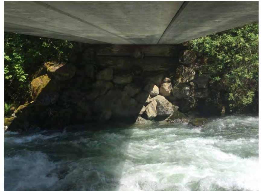
Right Bank Abutment when facing downstream
